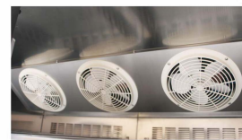
Fan-assisted evaporator and LED lighting
