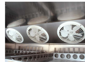
3-fan-assisted evaporator
